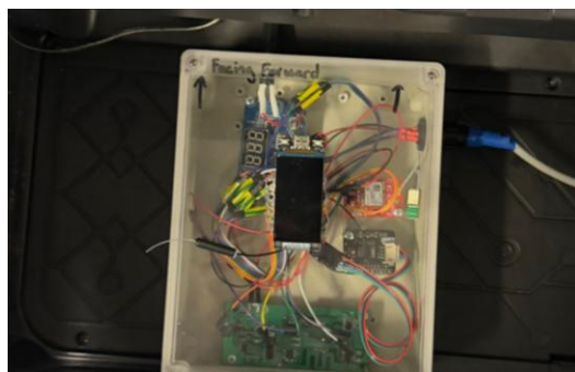
Figure 15: The Control box needs to have a forward-facing side due to IMU needing to know the corresponding direction of the car
